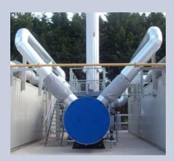
The Danstoker exhaust gas boilers for co-gen are plain tube single or twin-pass boilers, if necessary with an integrated economizer or superheater.
