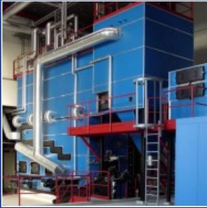
The Danstoker horizontal and vertical bio-fuel boilers are fire-tube boilers, and if required combined with water-tube sections. Capacities ranging from 200 kW to 50,000 kW or 68 t/h steam up to 43 bar-g.
